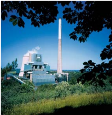
Evonik's Bergkamen Power Station
