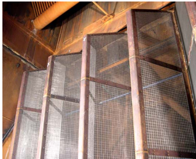
Separate filtering and structural support screens
