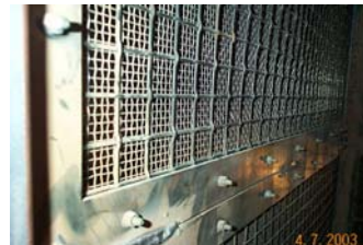
Separate filtering and structural support screens
