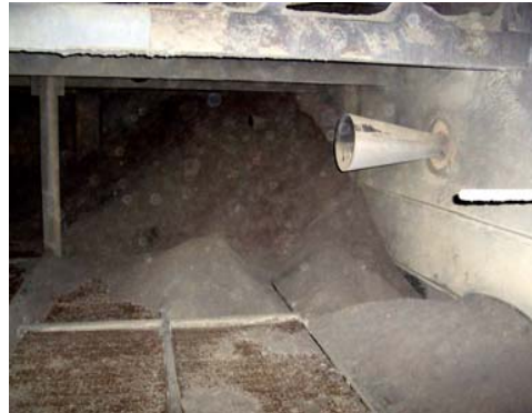
Fly ash accumulation on catalyst layer and pluggage
