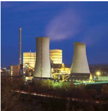
Evonik's Fenne Cogeneration Plant
